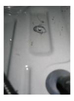
The inside hole can now be cut. Drill a 95mm hole around the hole centre.
